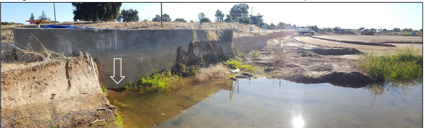
Photo of Cosumnes Irrigation Association diversion box next to Country Store with water leaking out from it and running into drainage with arrow indicating point of leak.
