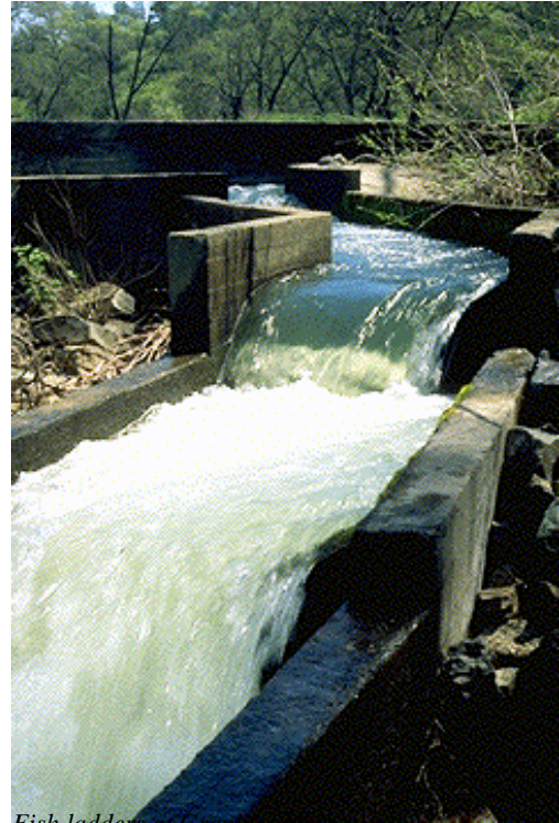
Fish ladders at Grantees Dam
