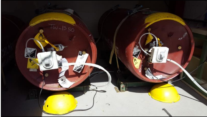
Ton cylinders of chlorine gas
