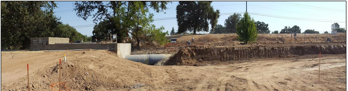
Photos of 42 inch pipe installed for Cosumnes Irrigation Association ditch on north side of Murieta Gardens
