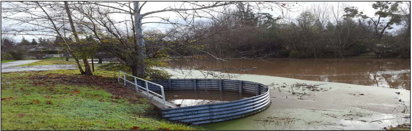
Basin 5 (Lost Lake) with water flowing through high flow trash rack outlet.
