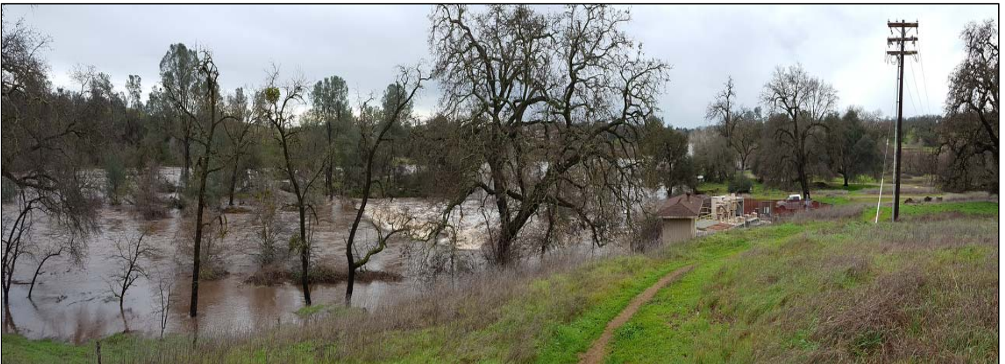
Granlees Diversion Structure, downstream view.
