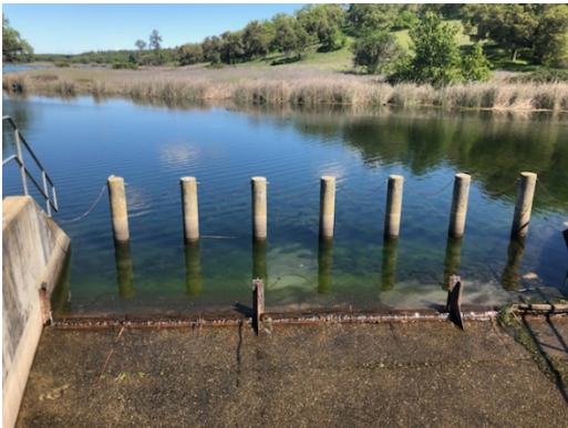
Photo of Clementia spillway 4/7/2020
