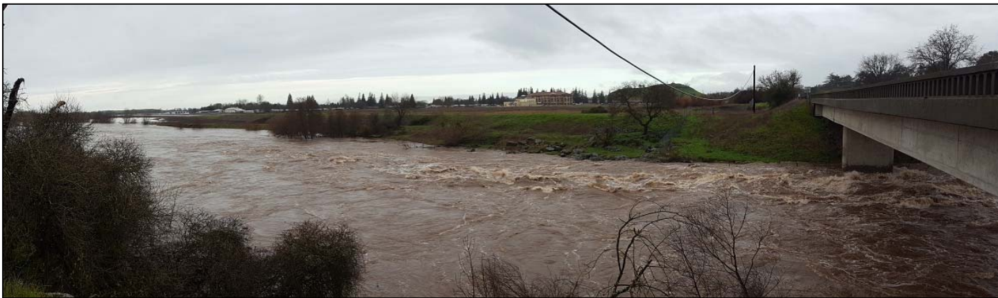
High flow in the Cosumnes River below the Highway 16 bridge, almost reaching up to levee 8068 (airport levee)
