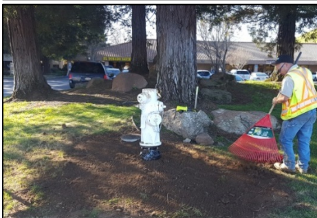
Utility Staff replacing hydrant
