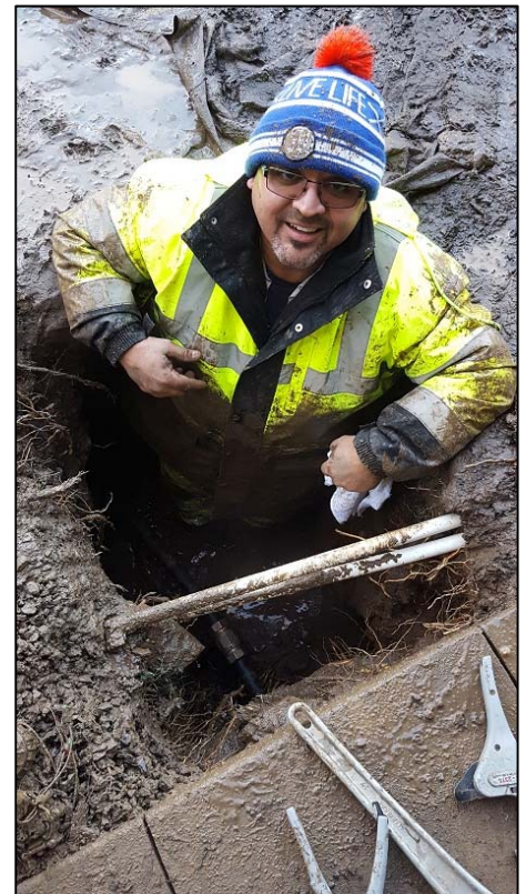
Service line repair at Murieta Plaza
