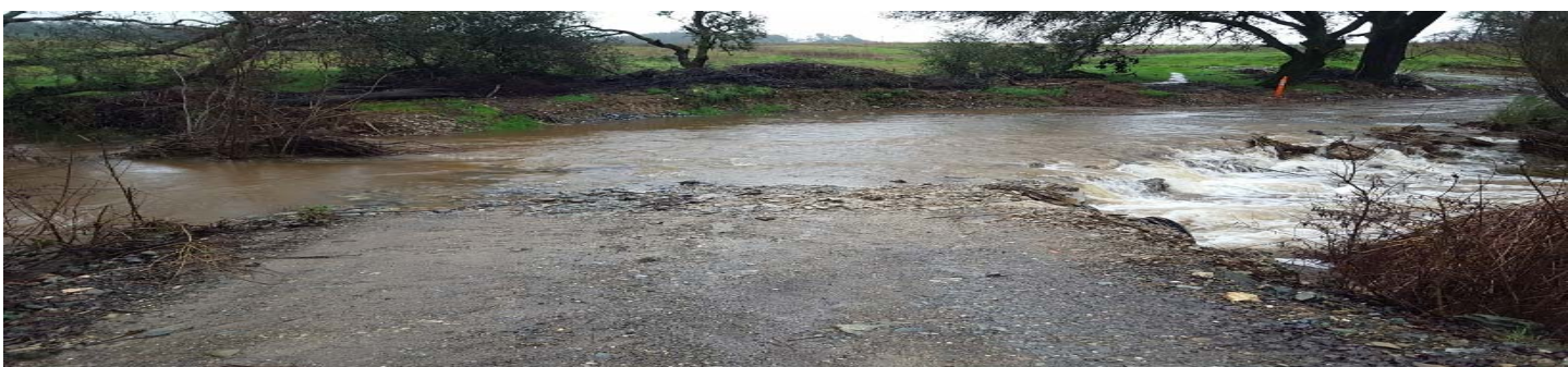
High flow across a Water Plant roadway after the storms
