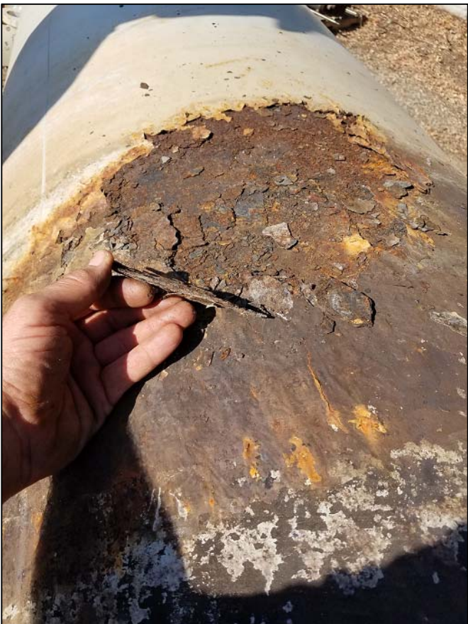
Corrosion of pipe column
