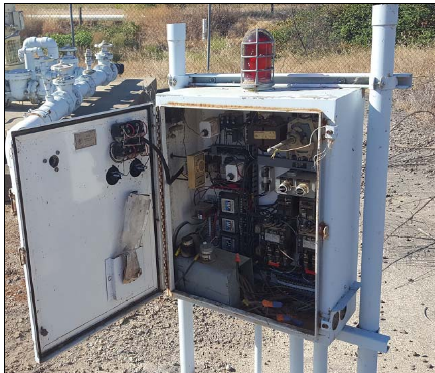
Photo of existing panel
