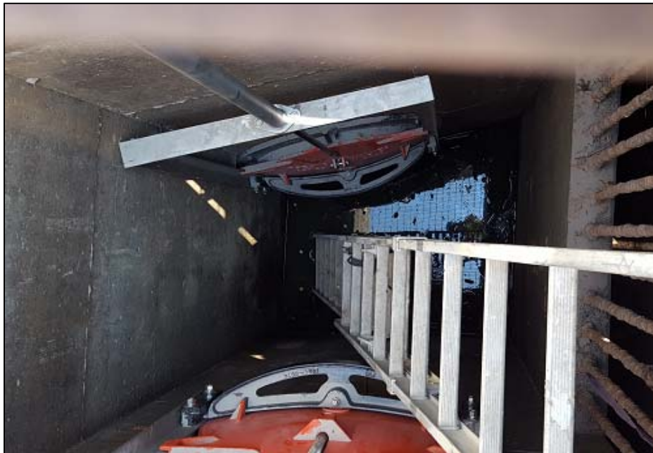
Two of the new sluice gates replaced at the Country Store diversion box
