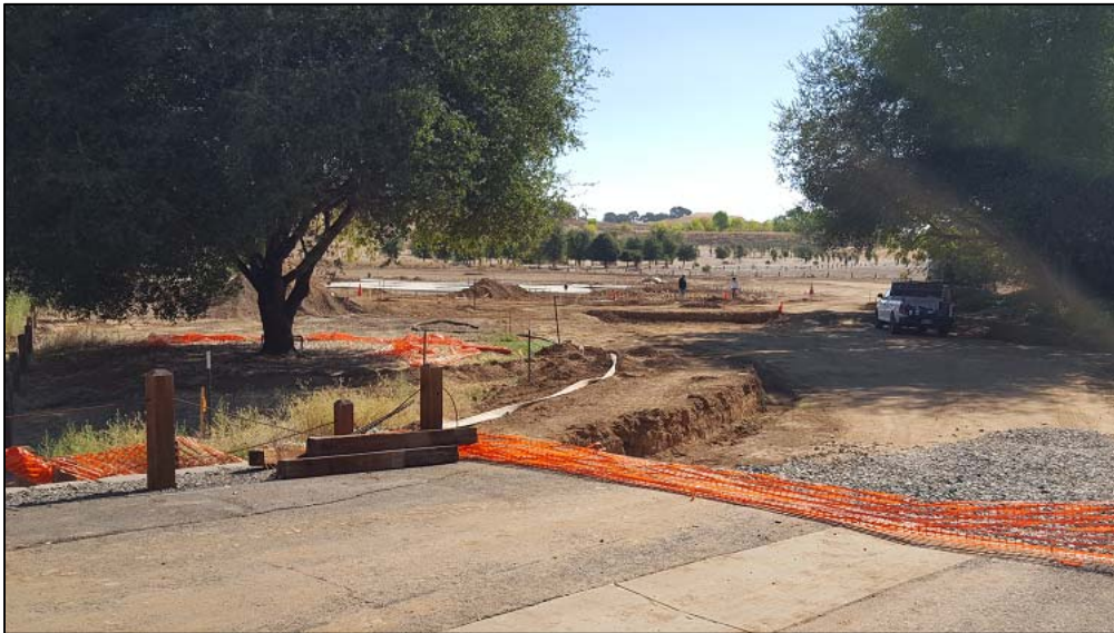
Greens Neighborhood Park under construction
