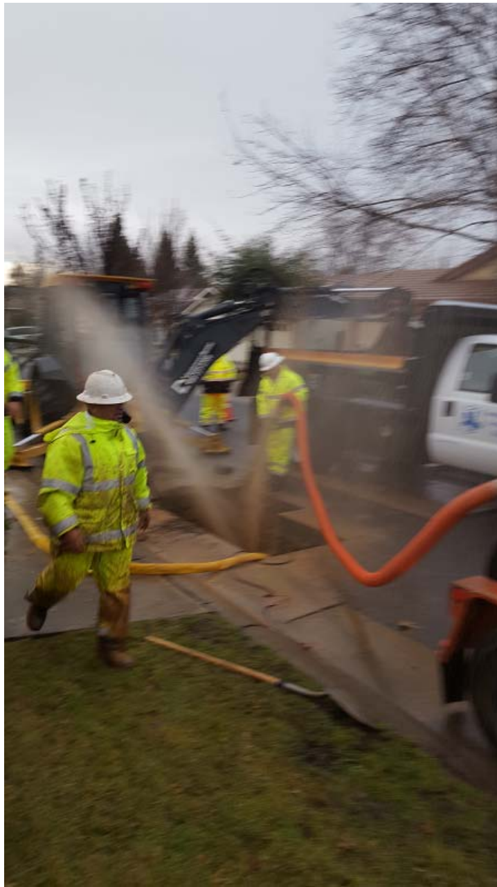
District staff working on Reynosa Drive water repair.
