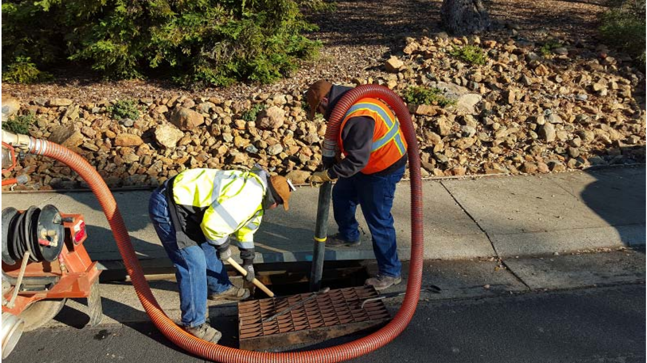
Staff cleaning debris out of a drop inlet (DI)
