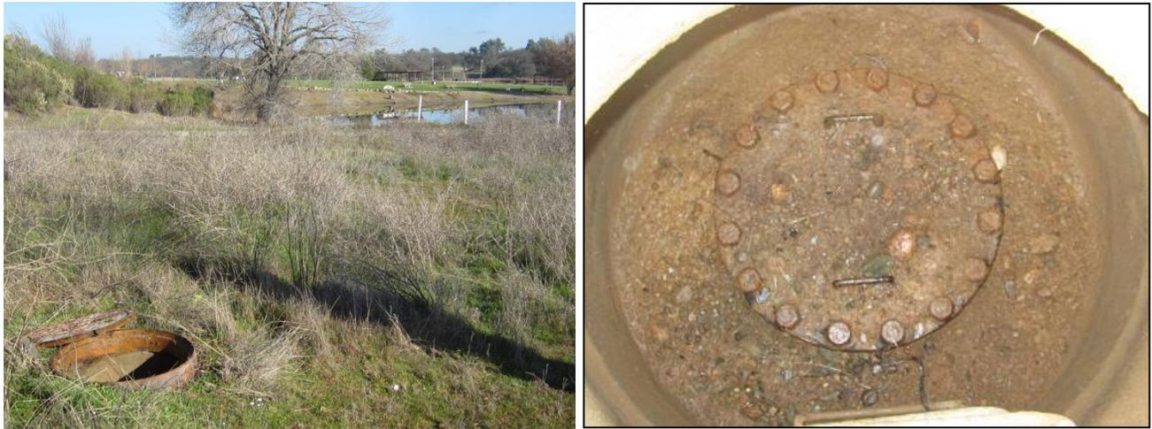
The 25" inspection flange will have to be adapted to accept the discharge flow from Clementia. A 25" to 12" concentric reducer spool will have to be fabricated and installed to receive a flange, Bauer or camlock fitting.
