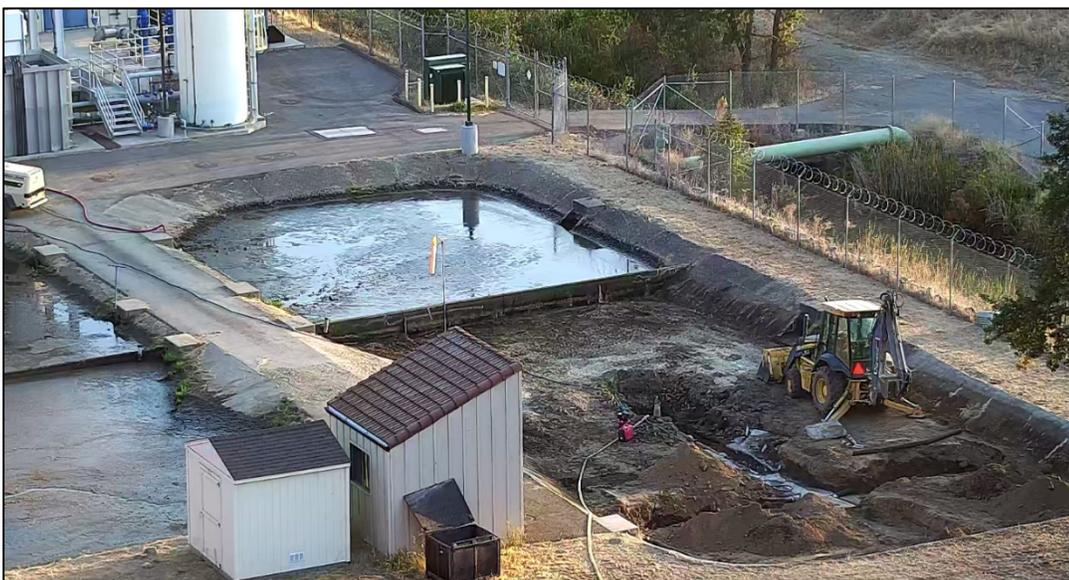
*Photo of drying bed piping being excavated*
