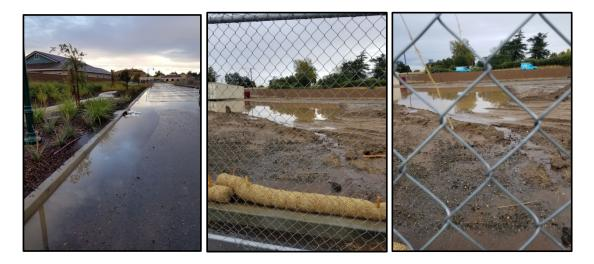
**The Retreats Project. P**roject BMPs implemented here are perimeter wattles, street DI perimeter gravel bags, and low point field silt fences. No construction activity has stared here yet. If anything some small large concrete pipe quantity has been delivery, and small construction equipment has been stage on site. My observation after the storm on this project has been of no issues all looks good since there is no ground disturbance.
