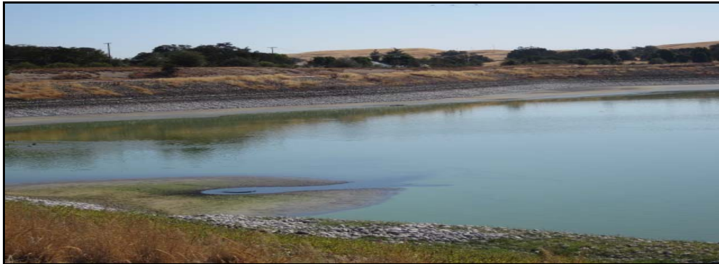
Secondary Storage Reservoir #1 showing influent structure exposed due to low level.
