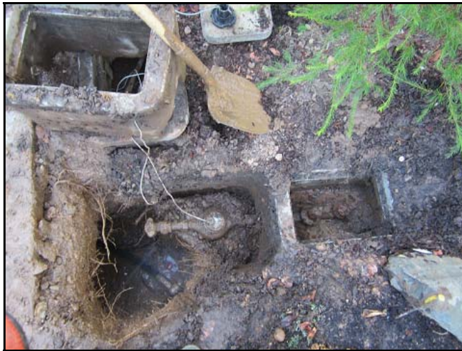
Water service line repair on Rio Circle.
