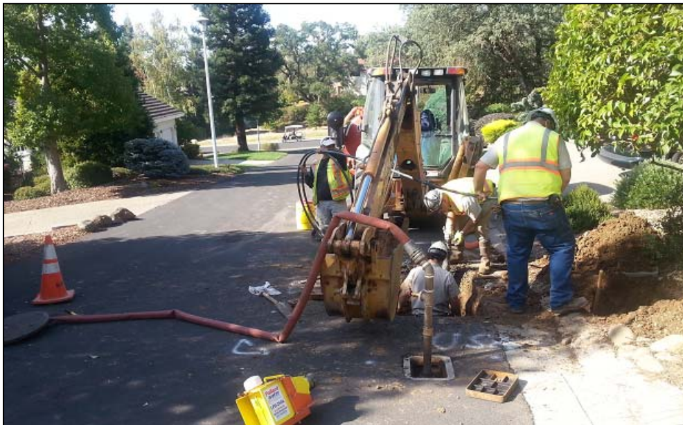
Utility Worker Jeff Hatfield, James Colas, and Jeff Nowell make a water line repair near Rio Blanco Drive
