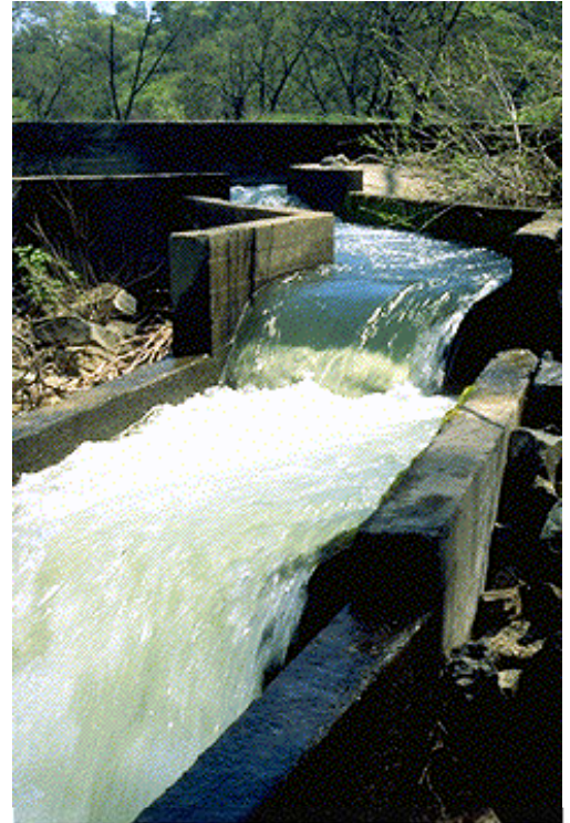
Fish ladders at Granlees Dam
