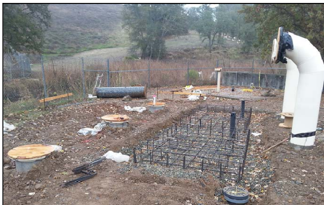
Forming of concrete pad for future raw water screening equipment
