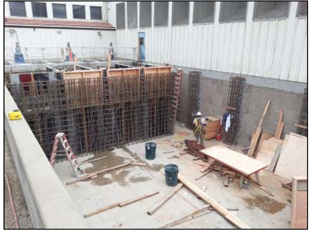
Forming of rebar for future membrane basins and setting forms for concrete to be poured
