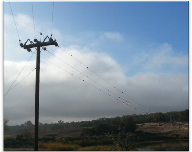
Reflectors put on power lines over Bass Lake.
