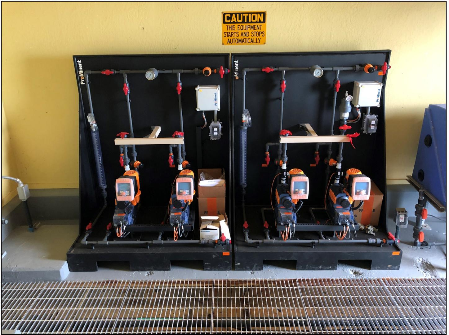
*Chemical feed skids placed in chemical feed room of Wastewater Reclamation plant*
