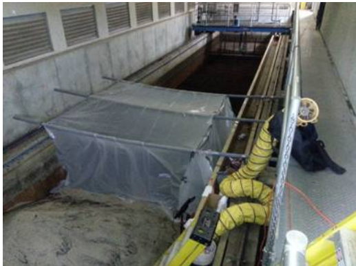
Photos of filter work being completed by staff.
