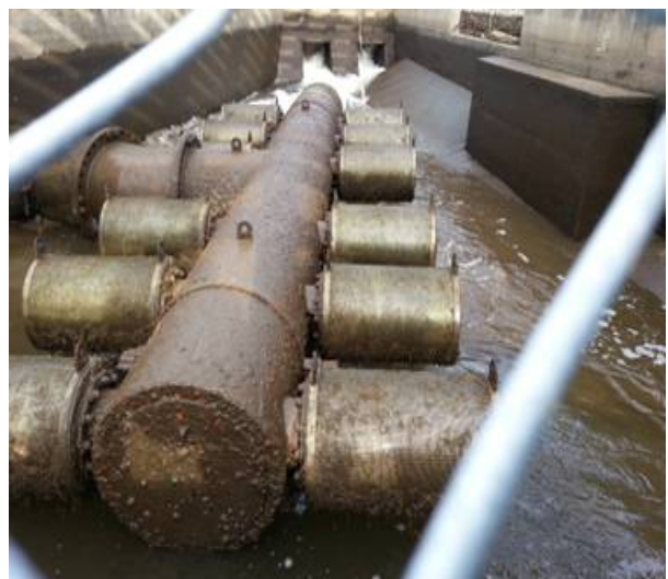
Photo of what the intake screens look like.
