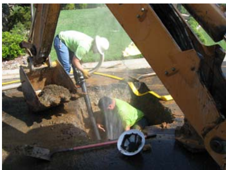
Water service line repair on Rio Blanco Drive
