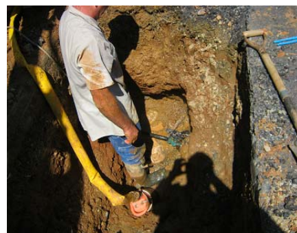
Water Service line repair at Medella Circle
